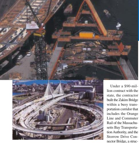
towers. In commenting on the bridge, the judges noted that it is visually striking, has well-executed three-dimensional detailing, and effectively utilizes high-performance (HP) 70W steel. They pointed out that the bridge's structural form was borne out of many functional requirements and stringent site constraints.
