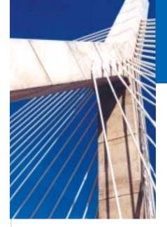
1,820 miles of steel wire were required to form the seven-wire strands that are in turn bound together to form support cables. The largest cables are up to 12 inches thick.
