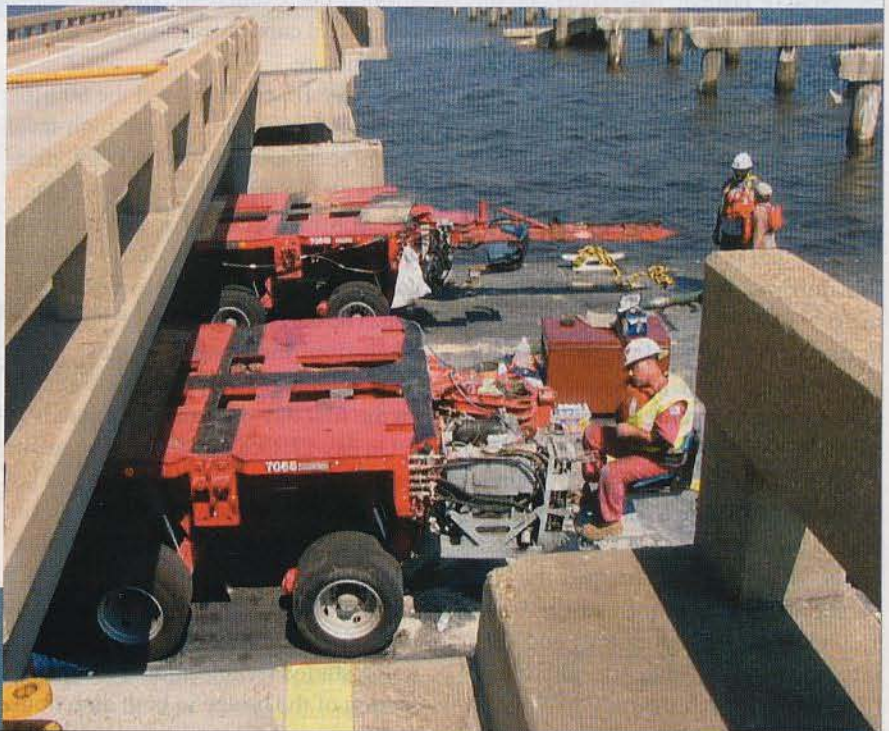
Specialized hydraulic Goldhofer platform trailers on a barge are used to lift and remove span 43 from the eastbound side. The span was moved and set into westbound Span 61.
