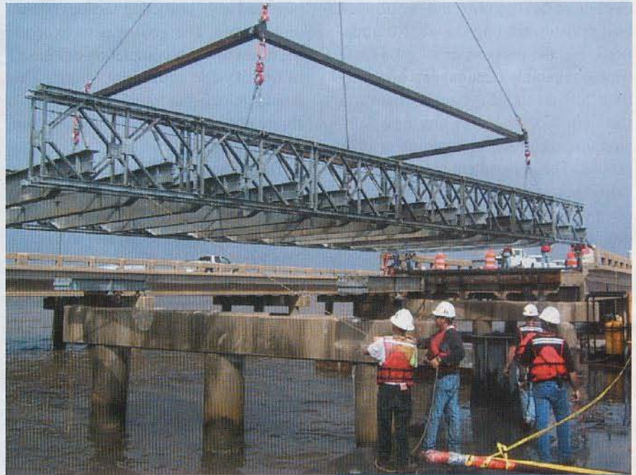
One of the 60-foot prefabricated steel Acrow bridge sections is lifted into place during the Phase 2 repair of the eastbound lanes.
