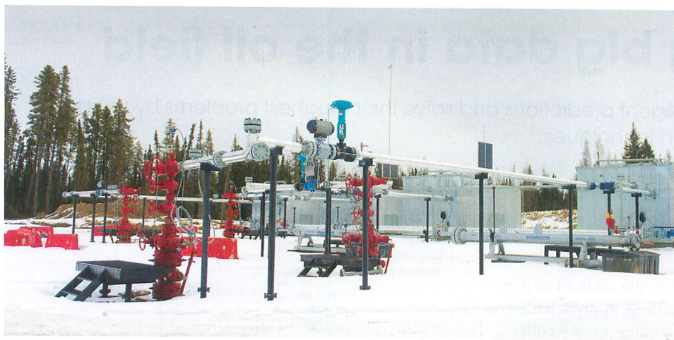
FIGURE 2. The well pads experience freezing temperatures for half of the year, so many well pad functions are contained in heated sheds (background), with one for each wellhead.
