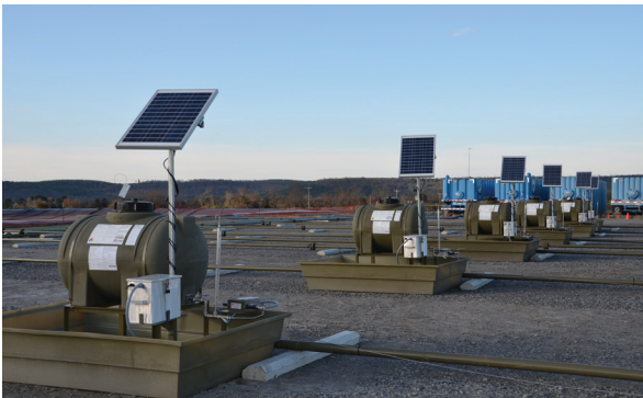
Solar chemical pumps are environmentally friendly and suit remote locations with limited or no power. (Photo courtesy of TXAM Pumps.)
