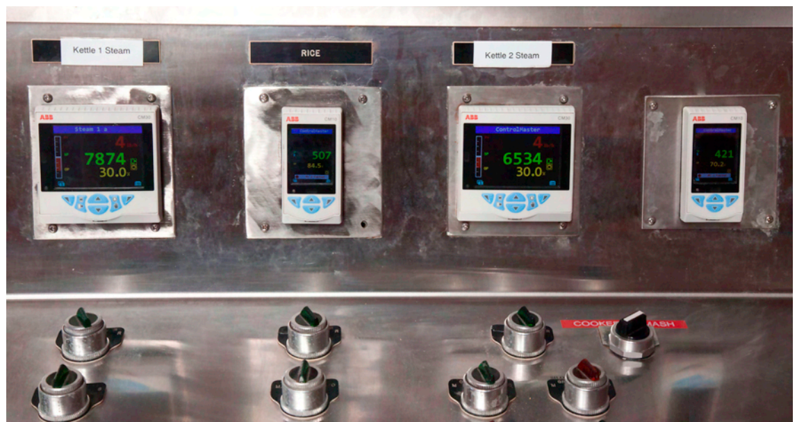
Control Panel containing the ABB CM30s and CM 10s.
