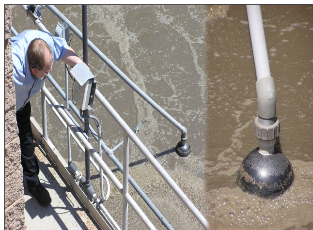
Figure 2. Dissolved Oxygen Sensor and RTD Sit Flush with the Bottom of a Large Floating Ball. Wastewater Flows Passed the Ball, Keeping the Sensors Free of Debris. Superintendent Mark Howarth Checks DO Reading on Nearby ABB Transmitter. The Transmitter Compensates for Temperature and Elevation and Sends a 4 To 20 MA DO Signal To The Control Room.
